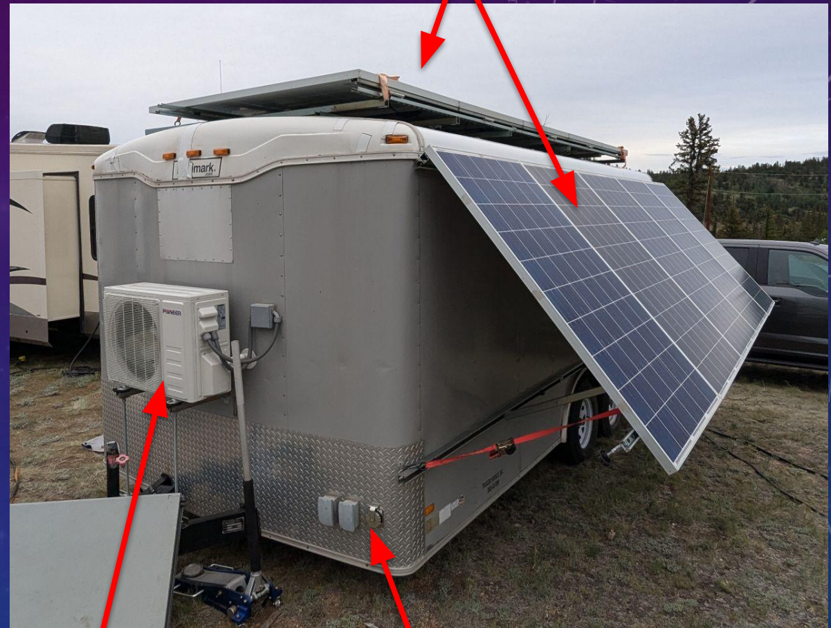
Mini-split heating and cooling
